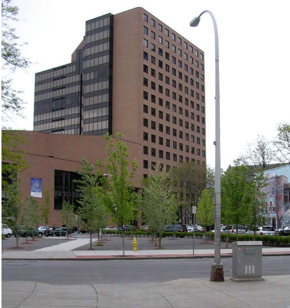
The Powelson Building site with the Civic Center in the background.
